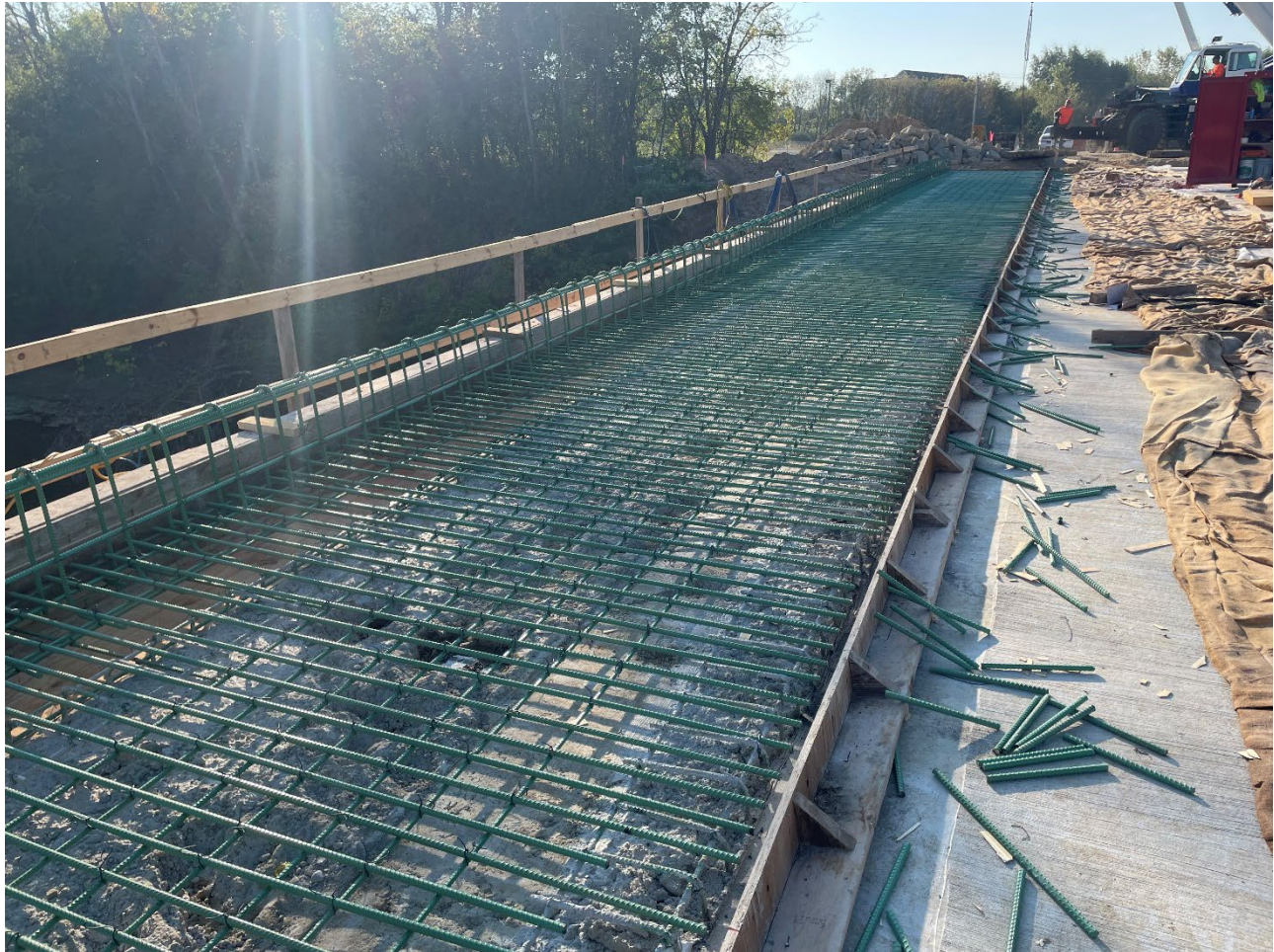
East sidewalk steel reinforcement and formwork
