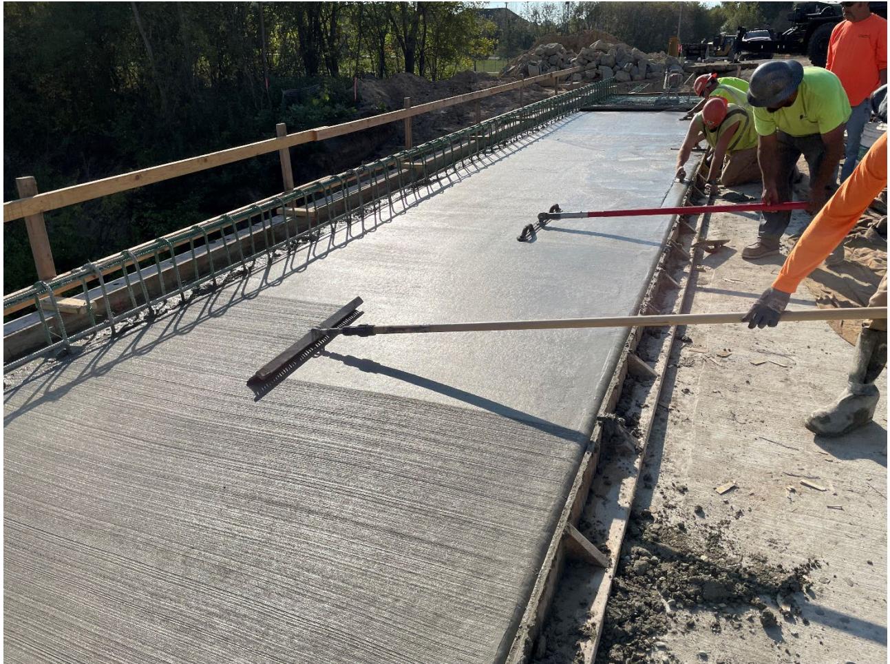
East Sidewalk smoothing and brushing
