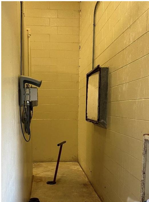
**Outside Air Louver with Motorized Damper, Dewatering Room North Wall**
