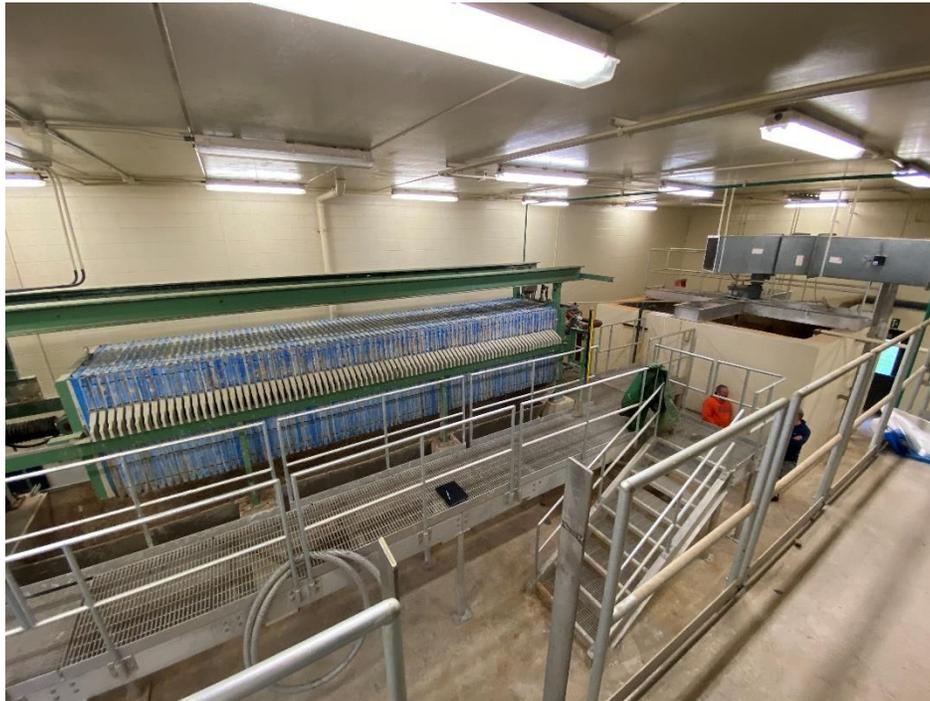
**Sludge Dewatering Room with Press on left and Reaction Tank on right**
