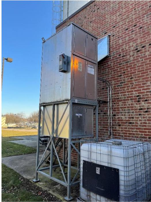
**Heating and Ventilating Unit, Vertical, Pad-Mounted**
