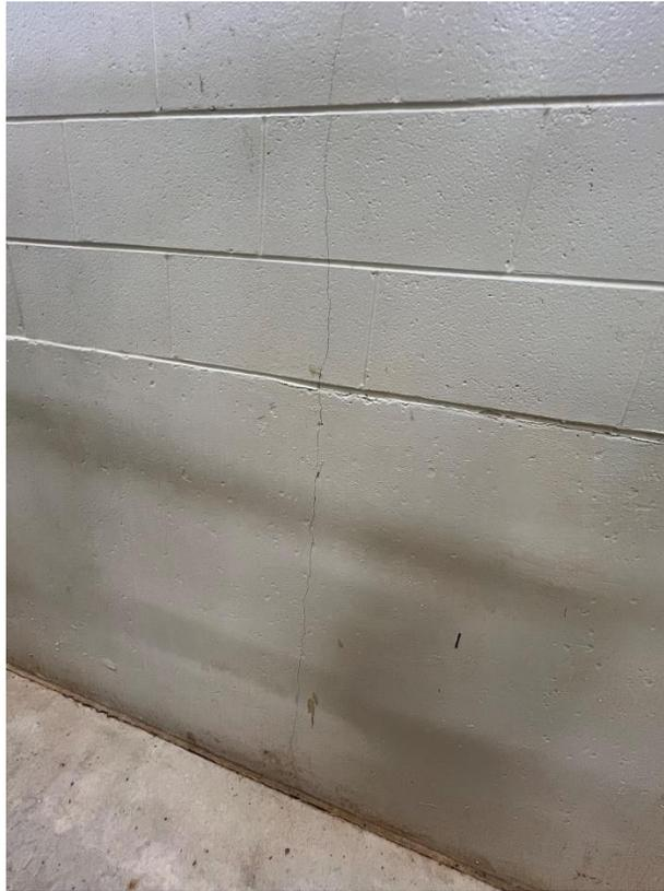
**Vertical crack in west wall CMU and cast in place concrete**
