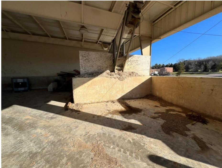
**Sludge Cake Storage Bunker and Screw Conveyor**
