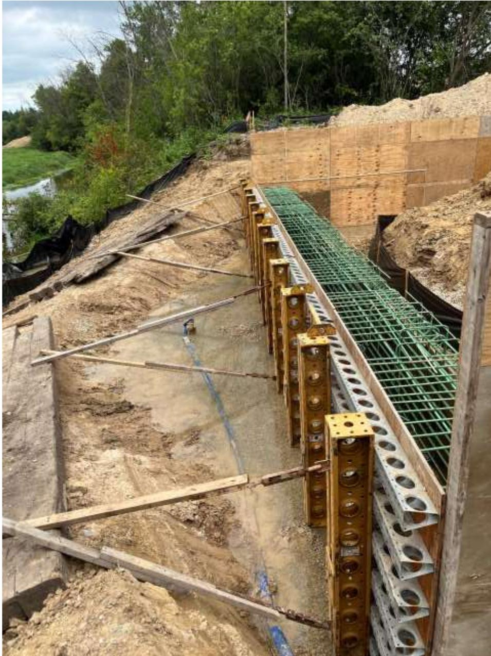
Installation of reinforcement within southern bridge abutment.
