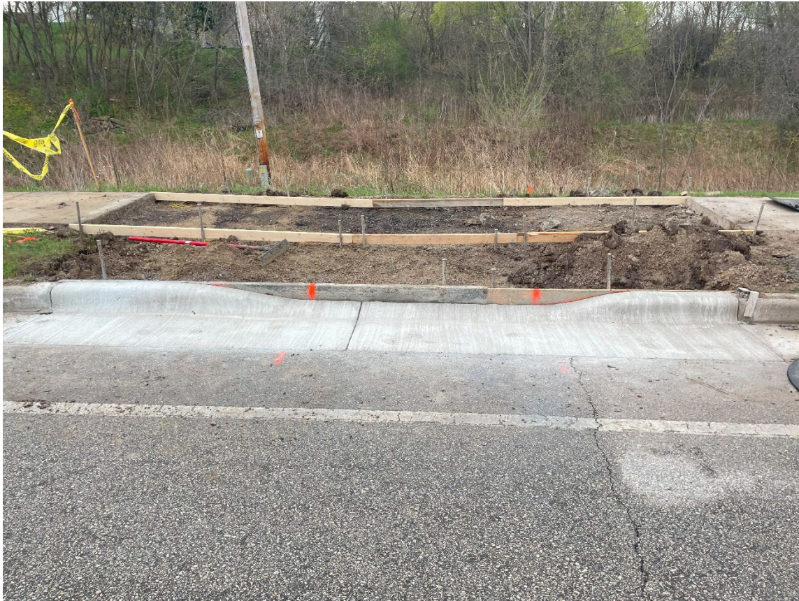
Ramp preparation on the south side of Aztalan Street.
