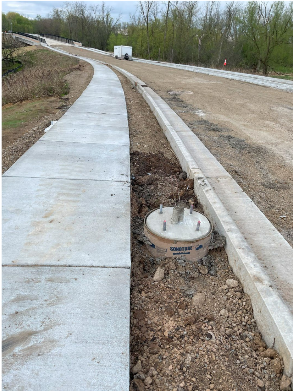
Electrical light pole base on north side of project.
