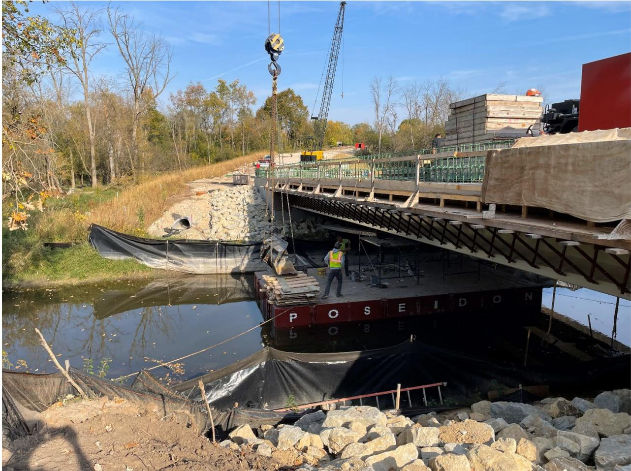
Stripping underside formwork on barge.
