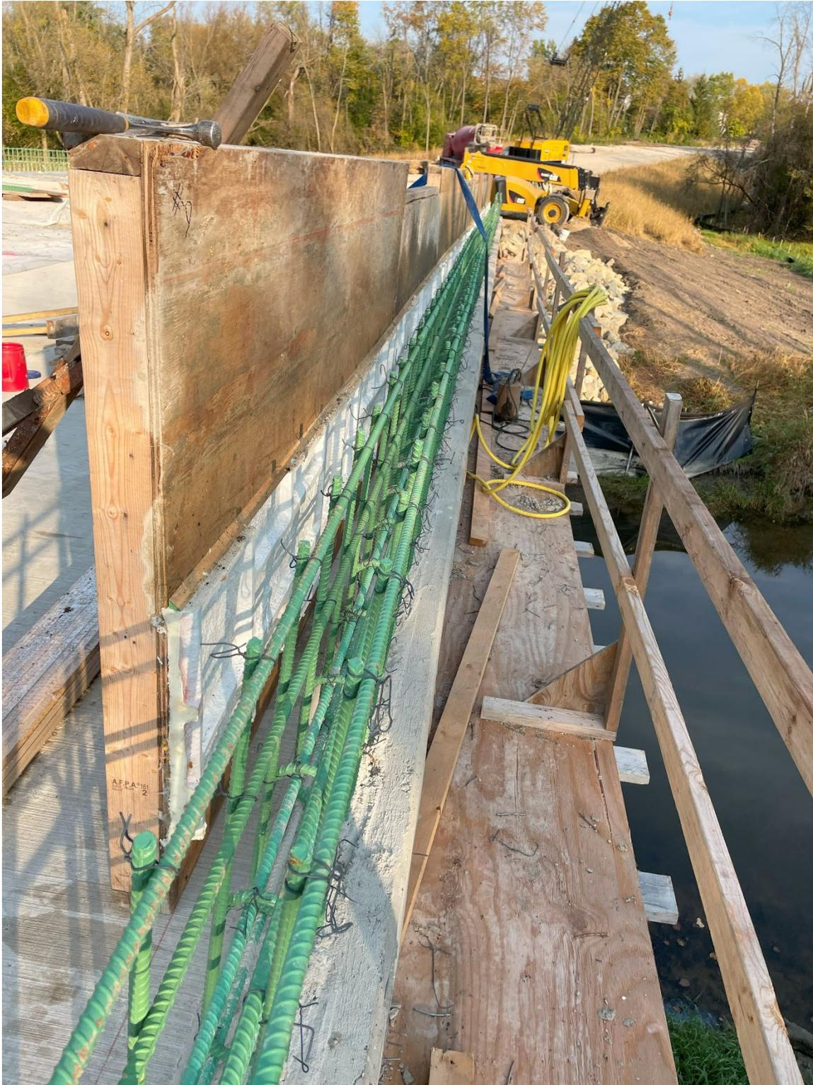
**Parapet steel reinforcement and formwork with rock form liners.**
