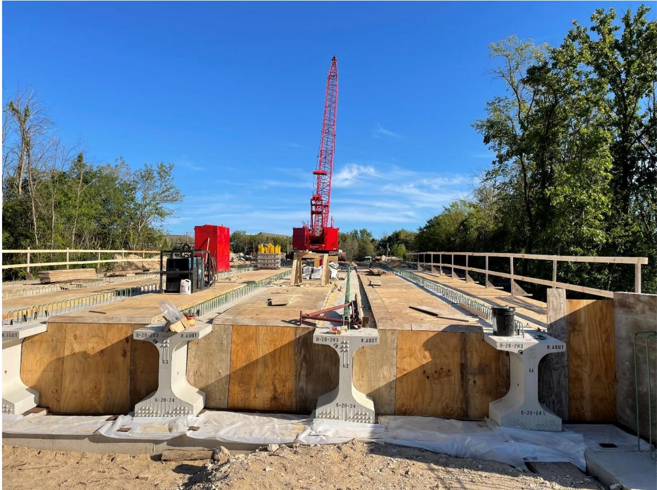
**Preliminary deck formwork with railings.**
