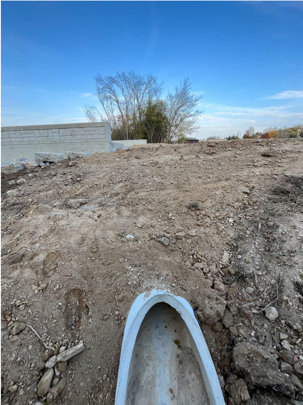
Final storm sewer outlet on south side of bridge.
