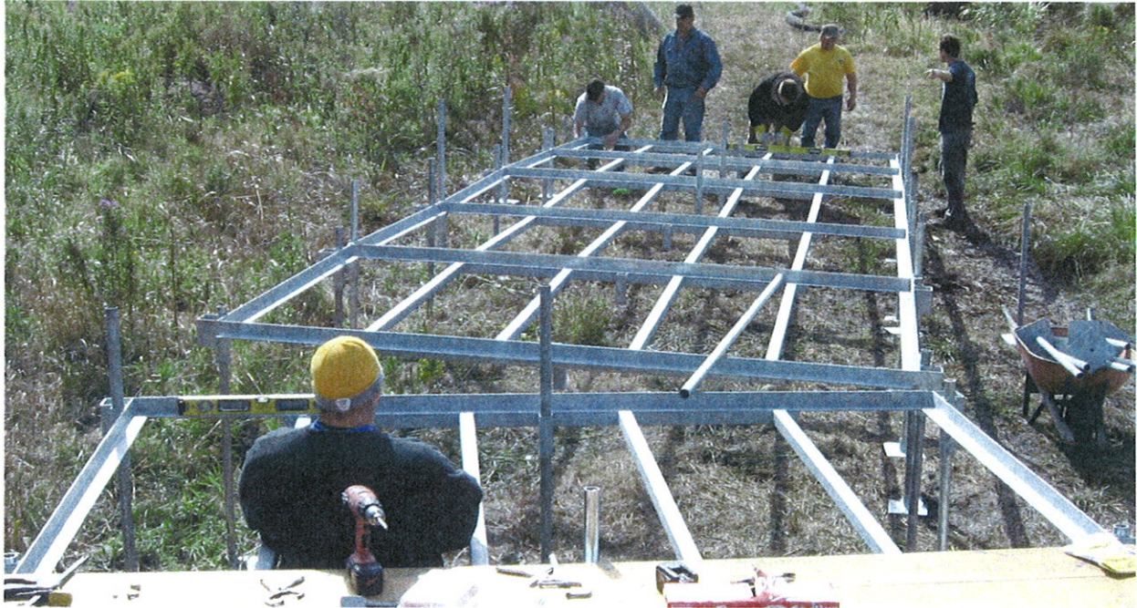
Image 11 – Boardwalk sections are easily constructed and geometry is almost unlimited – SAA 2009
