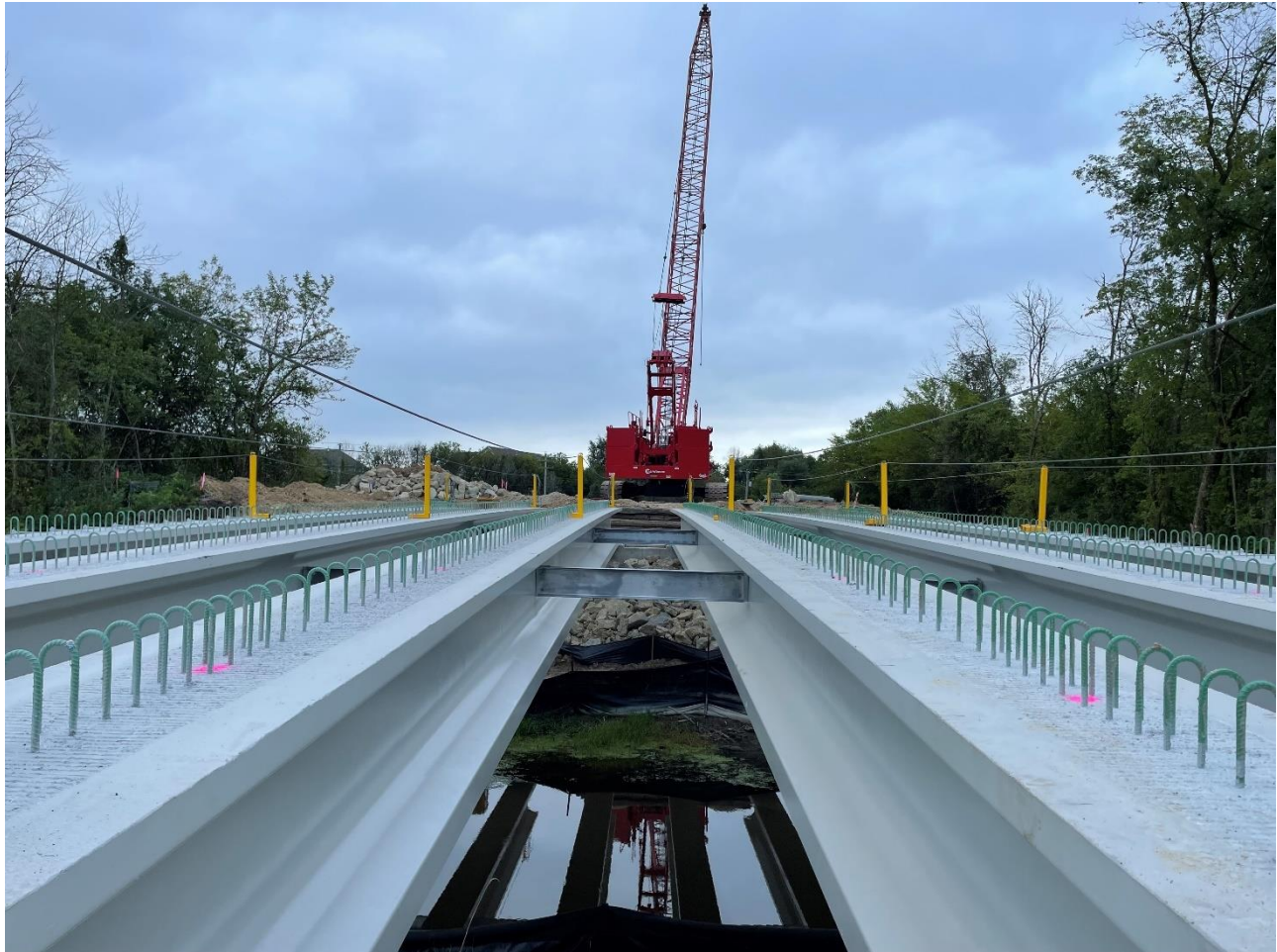
Installed girders from the north side.
