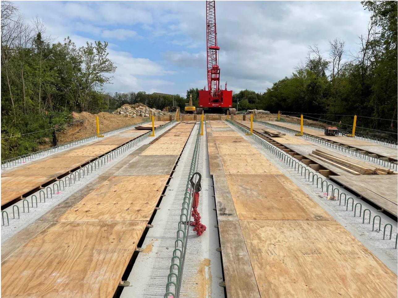
Preliminary deck formwork.
