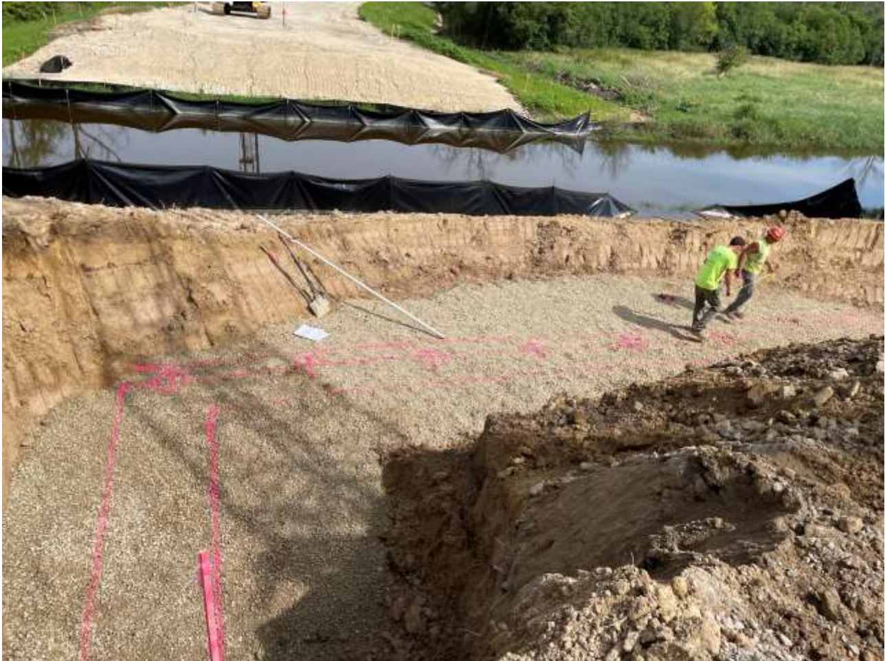
Southern abutment layout and excavation.
