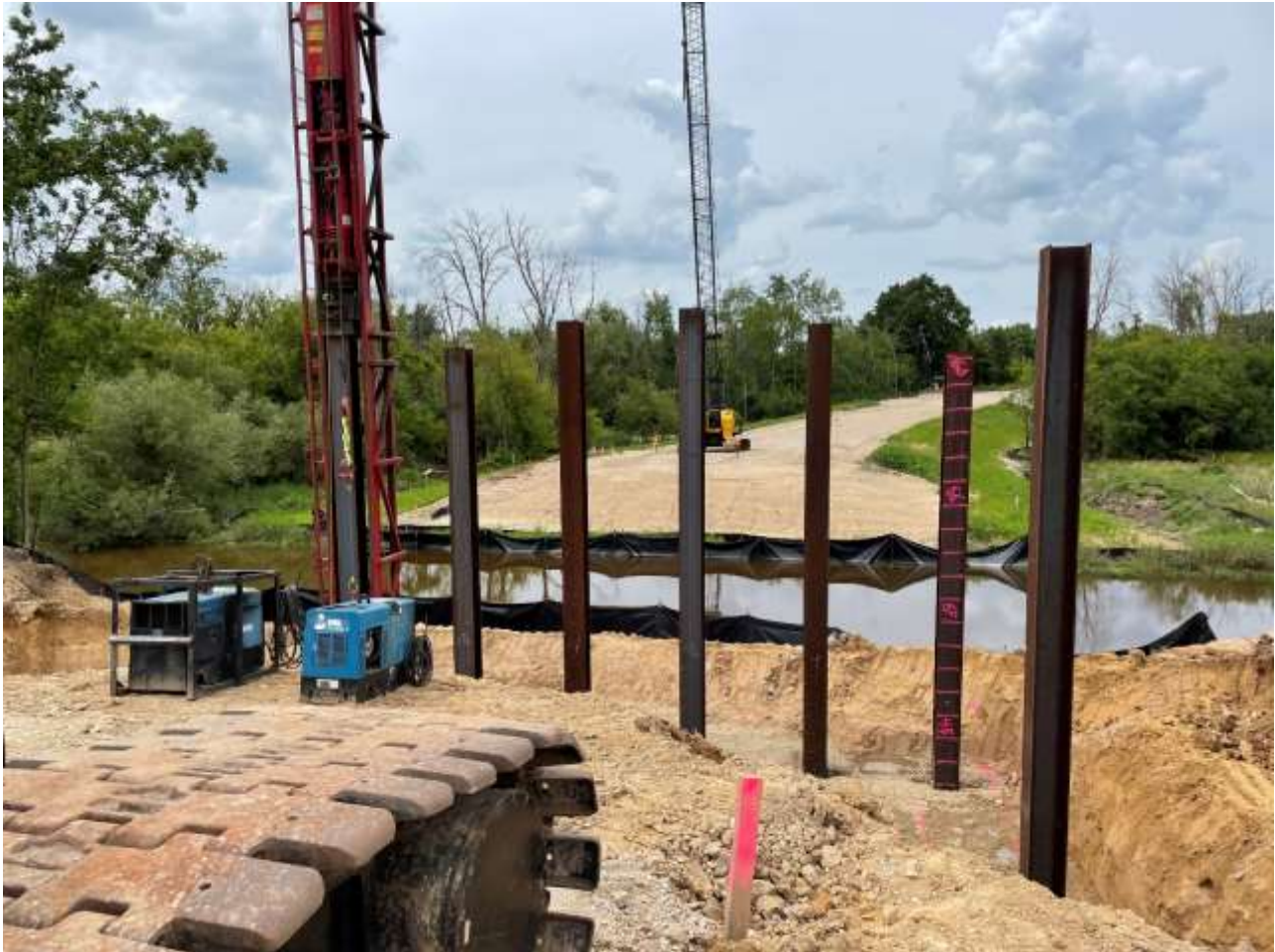
Pile driving on southern abutment.
