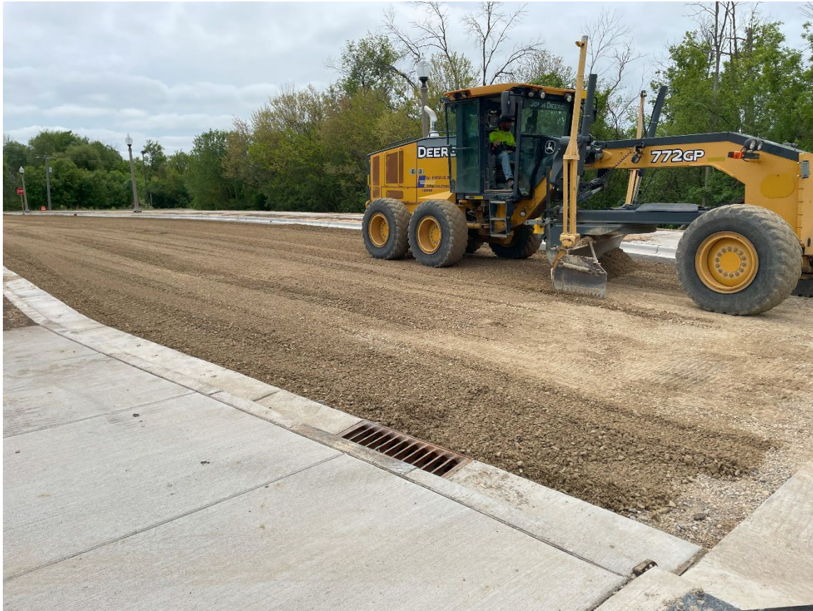
Fine grading of road subbase in preparation for paving
