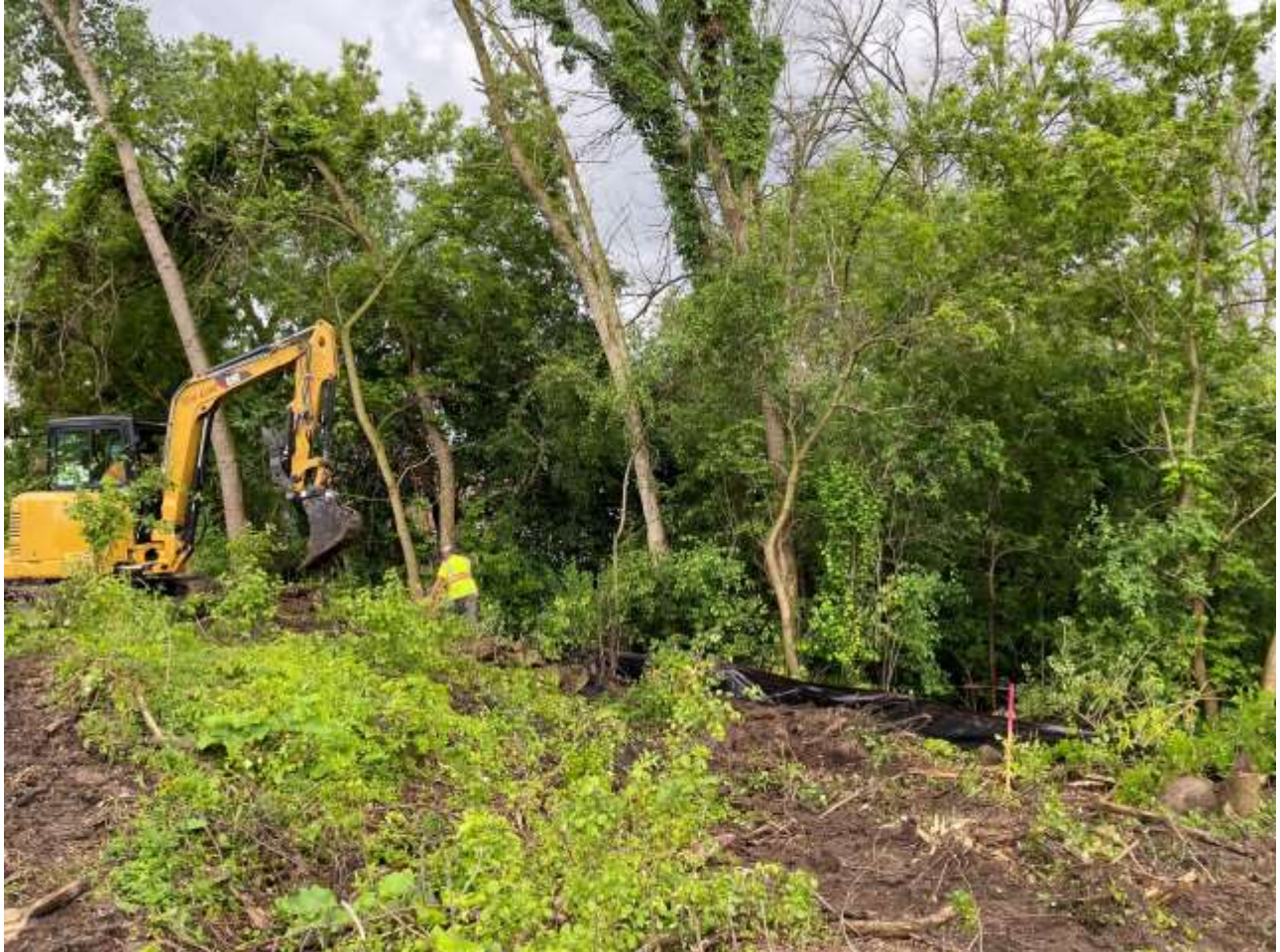
Silt fence installation in the flood storage area prior to excavation.
