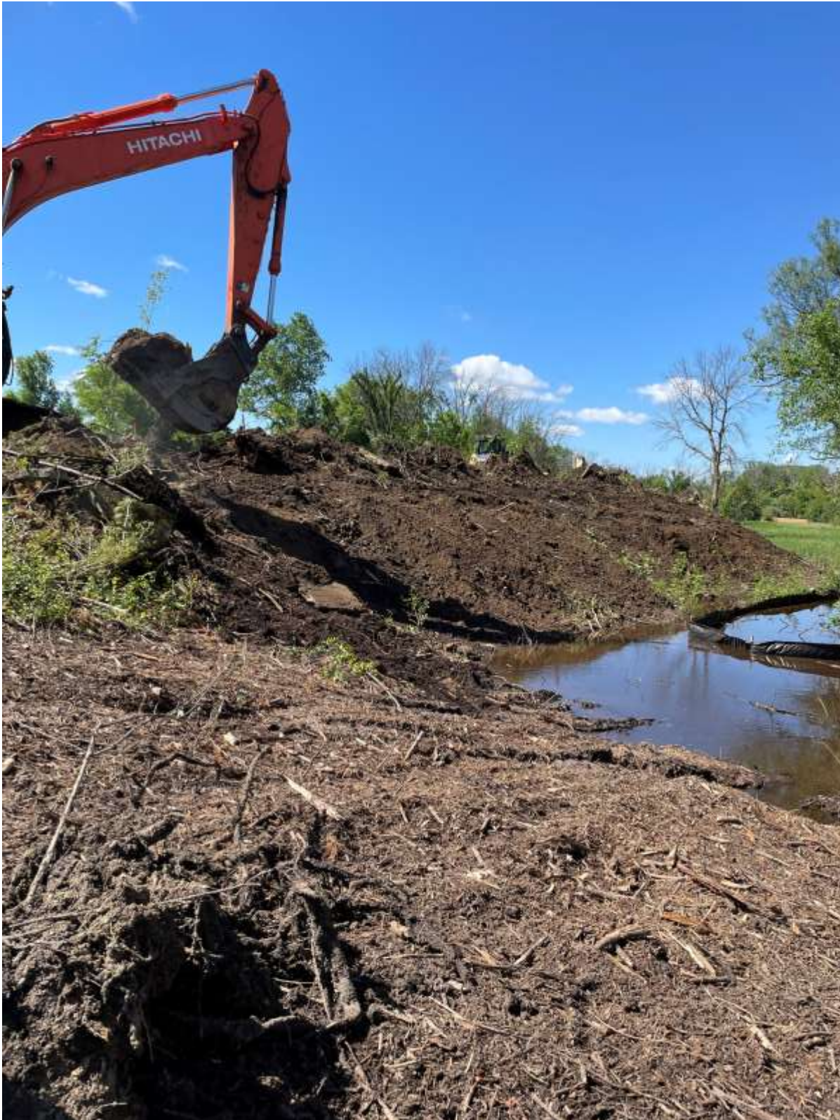
Excavation of the flood storage area.
