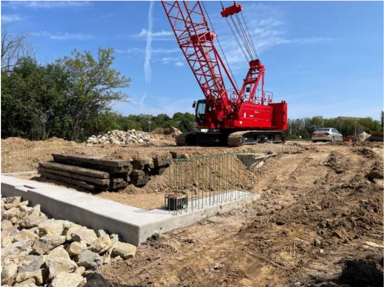
Southern abutment structure post-backfill and riprap installation.
