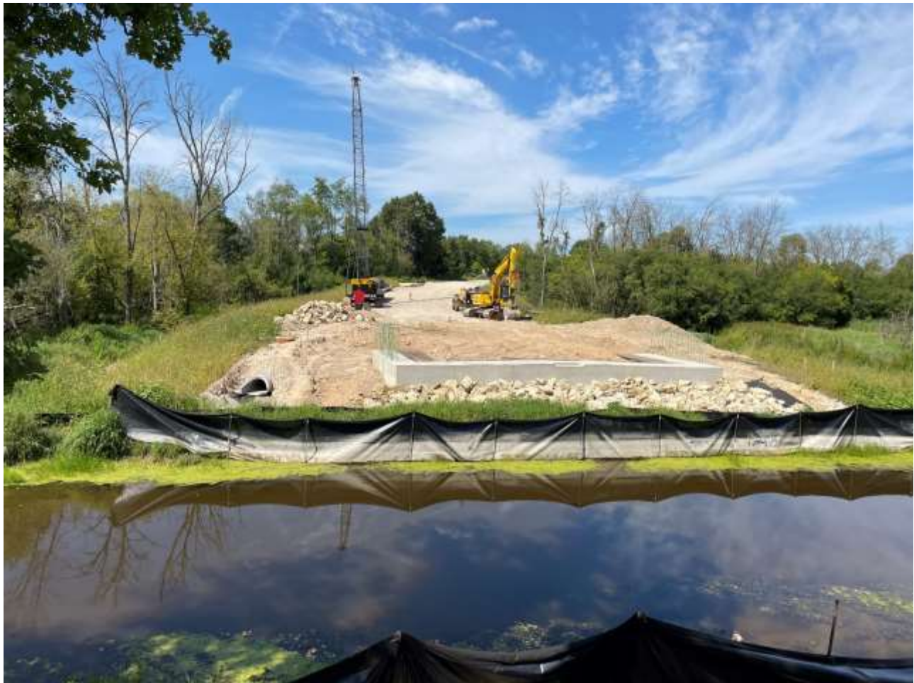
Northern abutment structure post-backfill and riprap installation.
