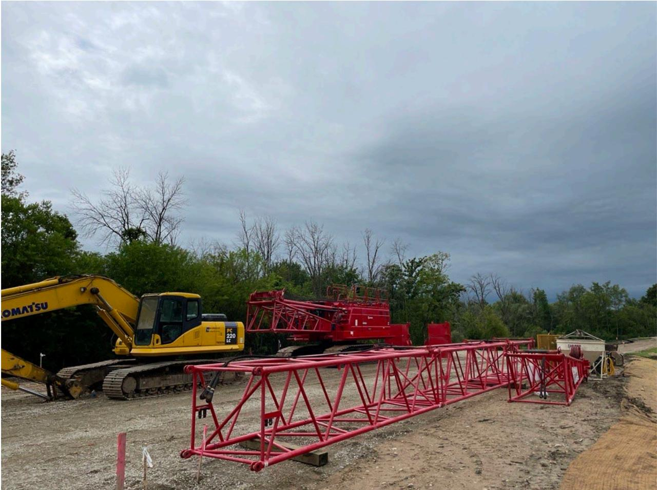
Disassembled crane in place on south side of the project in preparation for bridge construction.
