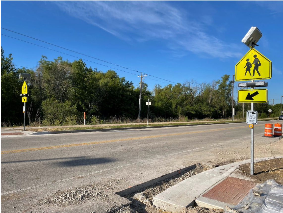
RRFB Flashing pedestrian crossing signs (not operational until road opening)
