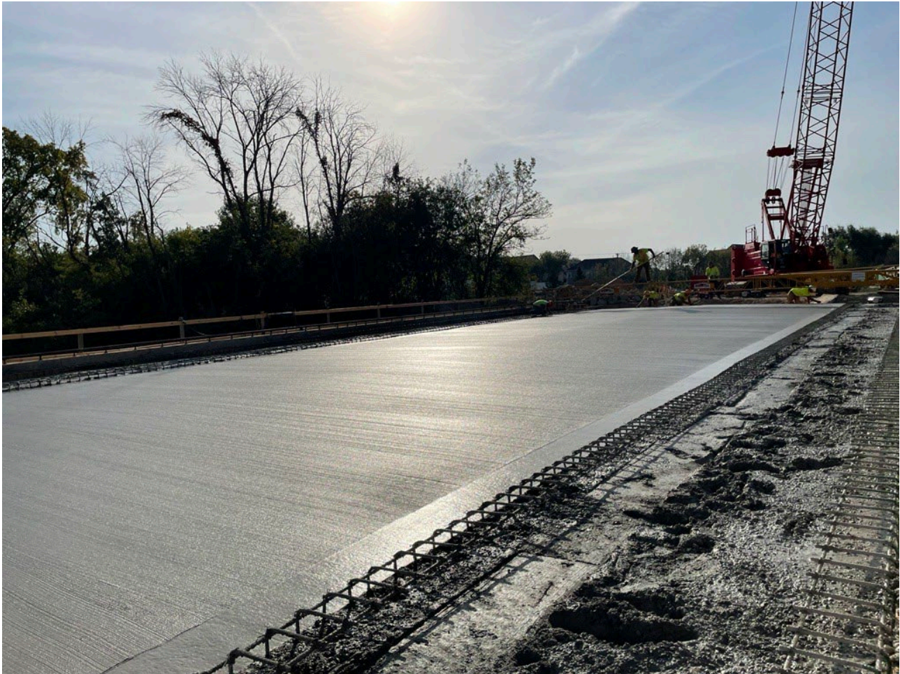
Finished Concrete Deck Before Curing.
