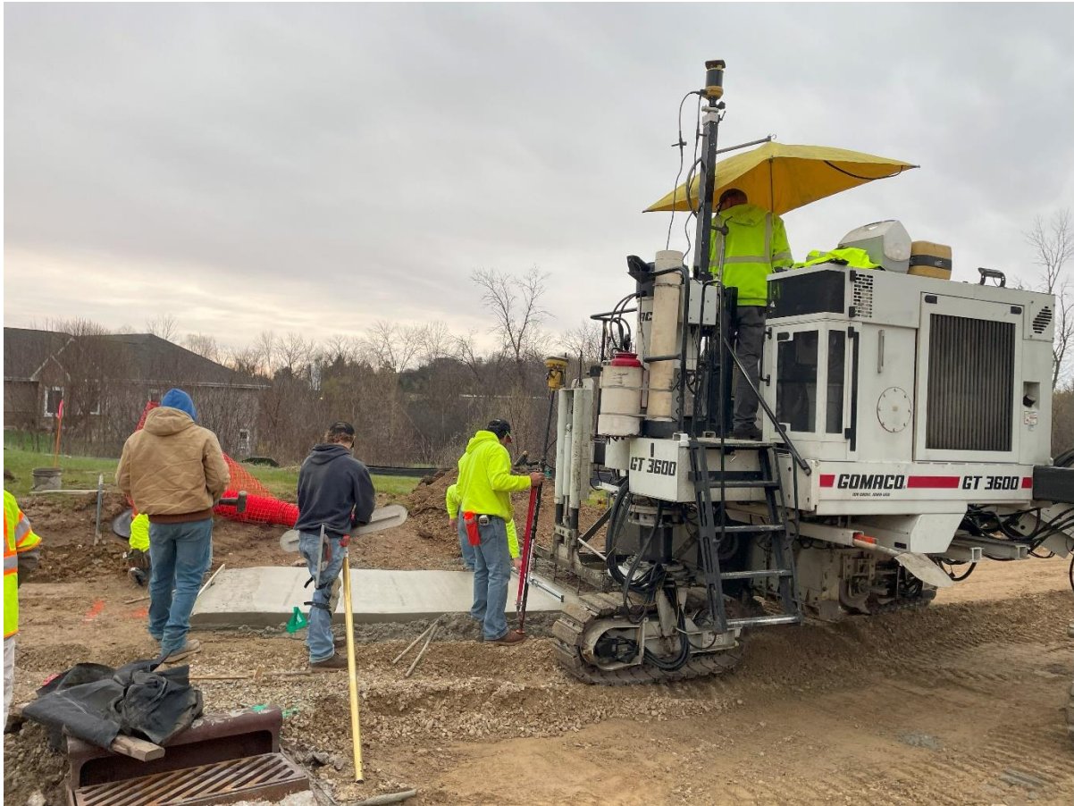
Schultz's curb and gutter machine installing sidewalk.
